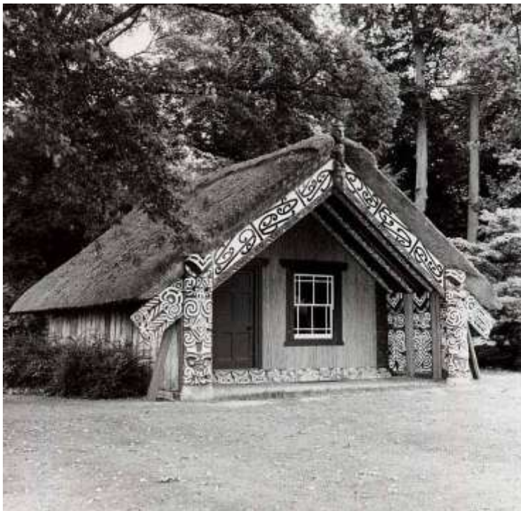
Hinemihi after restoration in 1980 (photo: National Trust Photographic Library).
